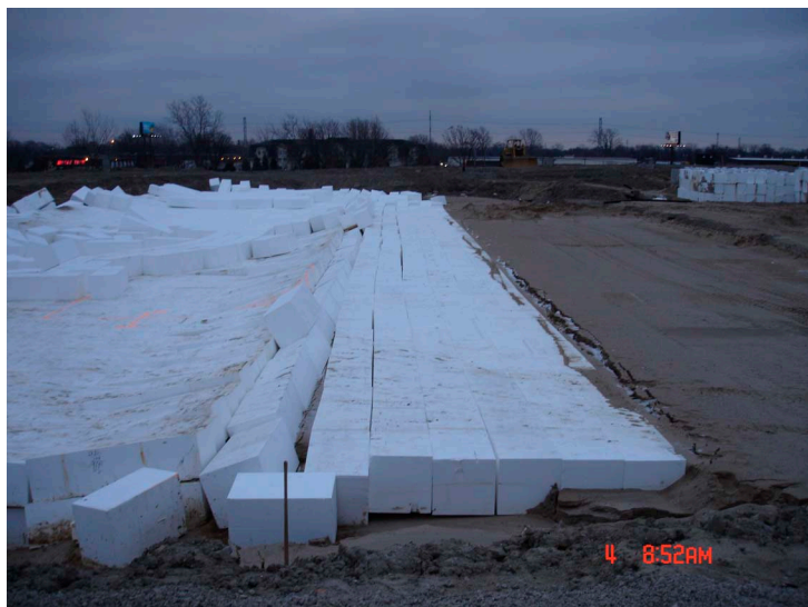
Figure 2. Ballasted edge of geofoam foundation
