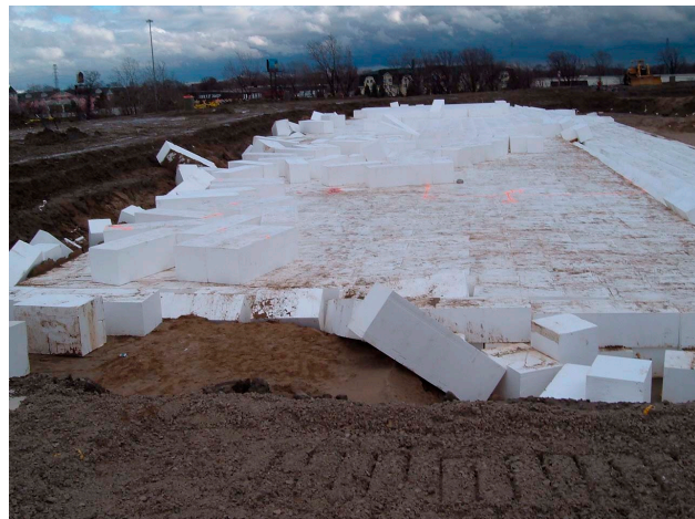
Figure 4. Incident site looking East
