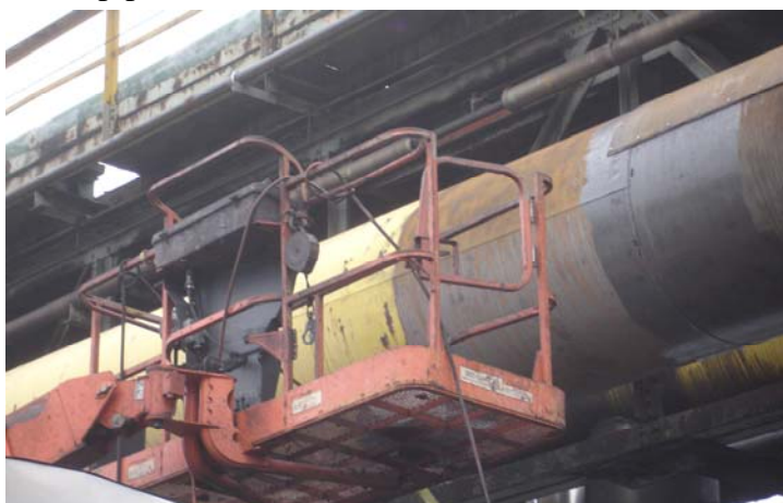
Figure 5. Gasketed steel cladding patches and man lift
