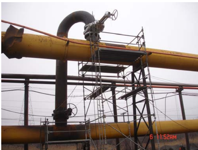
Figure 2. Example of bypass piping
