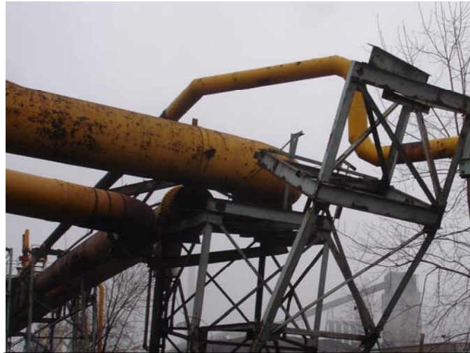
Figure 7. End of pipe where blank exited
