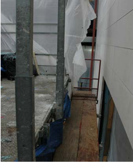
Figure 5. Guardrail installed on north end of working plank after incident
