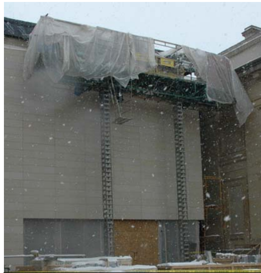
Figure 2. Repositioned Hydro Mobile 2 scaffold
