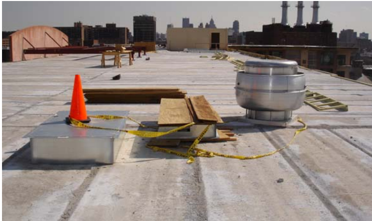
Figure 1. Make-up air roof curb with orange pylon, exhaust fan roof curb with plywood, looking south on roof
