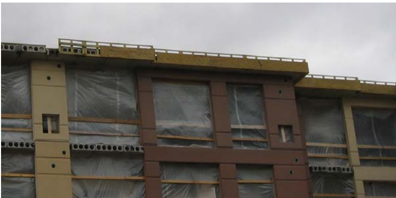
Figure 6. Example of parapet work construction
