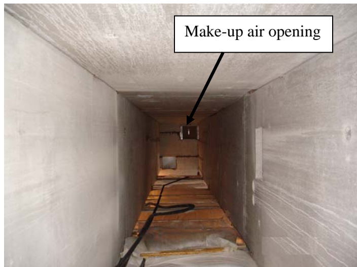
Figure 8. Chase A openings as seen from the basement, facing east
