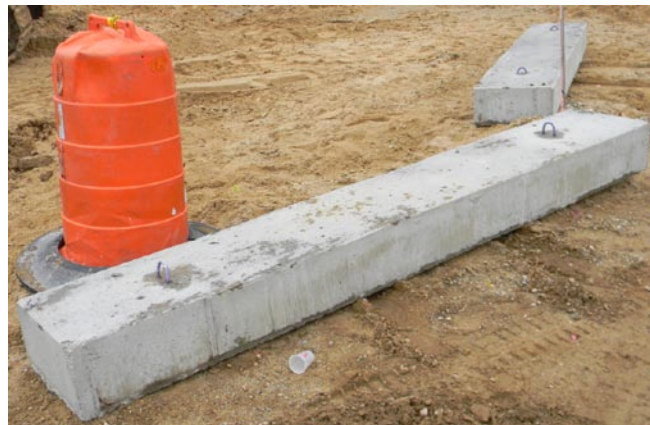
Figure 2. Concrete deadman anchors used on east and west sides of trench
