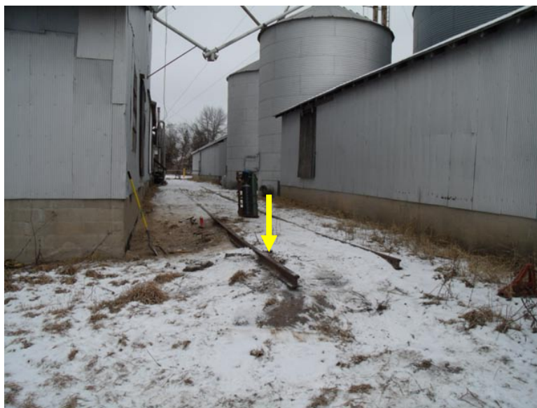
Figure 2. Identification (yellow arrow) and location of railroad spur being removed
