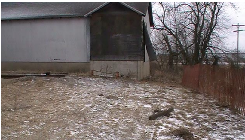
Figure 3. Overview of incident site after incident. Note orange fence installed by employer at embankment edge.
