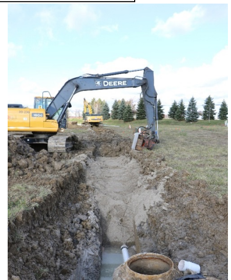
Figure 2. Water location in trench
