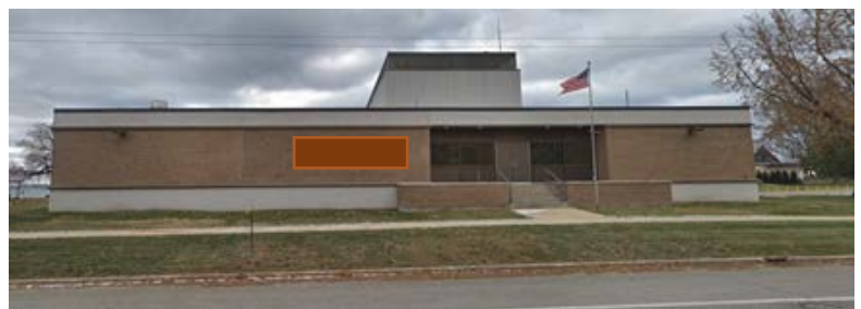
Photo 1. Front of water treatment plant undergoing renovation.
