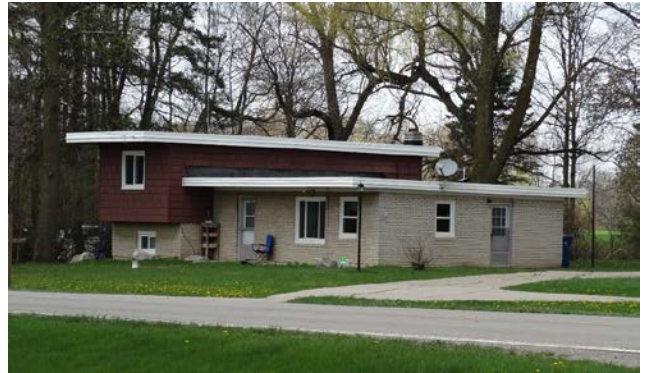
Photo 1. Picture of home where decedent was siding. Decedent working on lower level flat roof.
