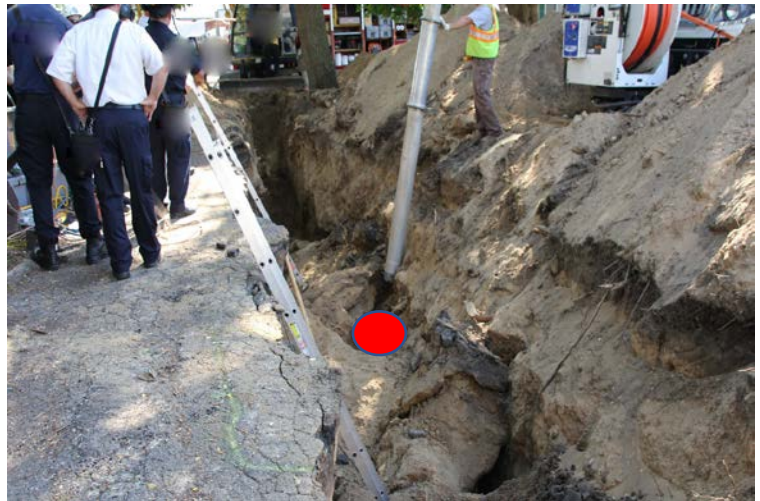
Photo 4. Vacuum truck removing soil from around decedent. Red circle is location of decedent.
