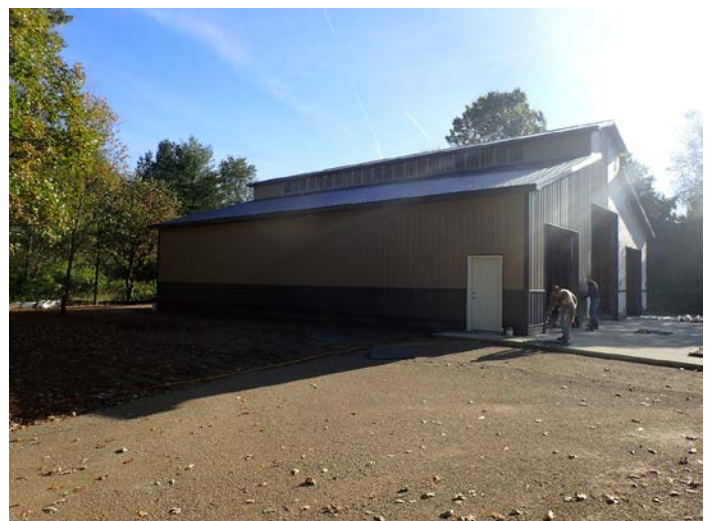
Photo 1. Pole barn under construction
