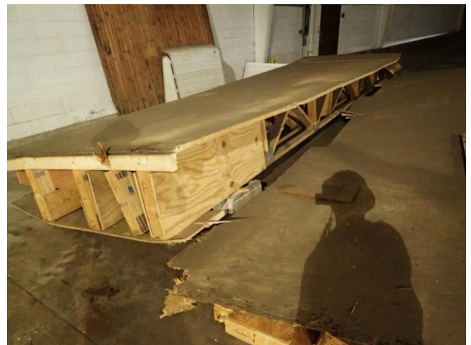
Photo 2. Example of truss/floor joists with foam-covered plywood that had previously been removed.
