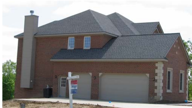
Figure 3. Side view of home under construction
