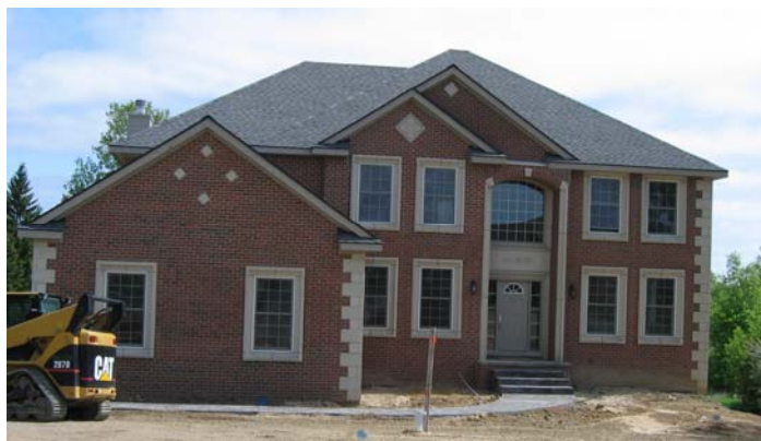
Figure 2. Front view of home under construction
