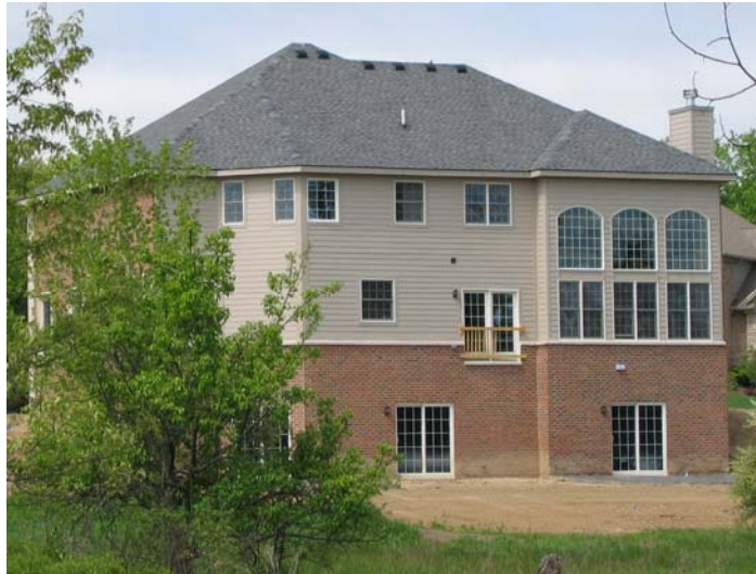
Figure 1. View of rear of residence under construction
