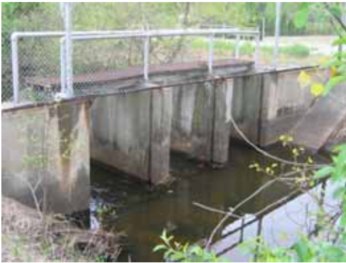
A male farmer, who was a member of a volunteer cooperative drowned, as he was removing wood stop logs from the drain's water level control structure to relieve a high upstream water level. MIFACE Investigation 08MI135
