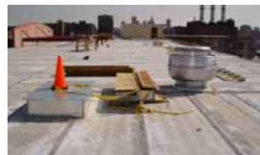
A male construction worker fell from the roof of a five-story building through a 26-inch by 24-inch make-up air opening of an elevator shaft to the concrete floor of the basement. MIFACE Investigation Report 08MI015
