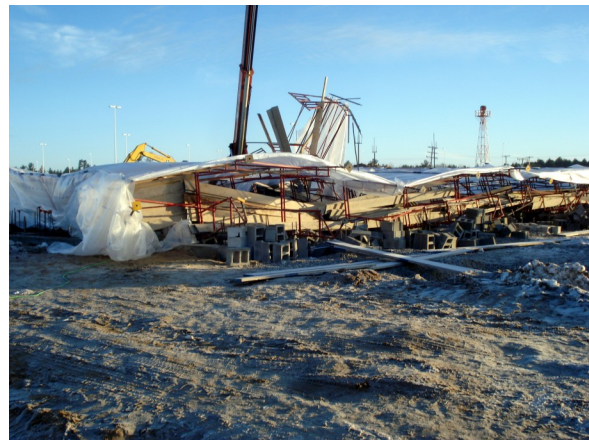
Brick mason died when scaffold collapsed while erecting wind screen
