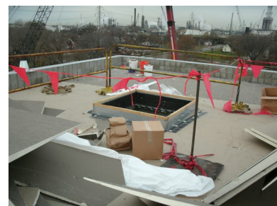
Hispanic roofer fell through improperly protected roof curb
