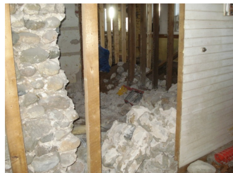
Carpenter died when a basement's stone wall collapsed
