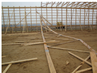
Building contractor died from 30-foot fall when an 82-foot long truss collapsed
