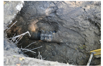
Gas utility worker died due to asphyxia while repairing a 6-inch cast iron natural gas line
