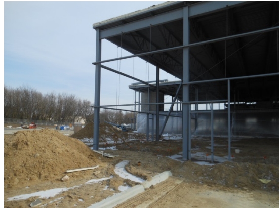
Case 15. Male roofer fell approximately 26 feet when the cantilevered 2" rigid roof insulation he stepped on broke away.
