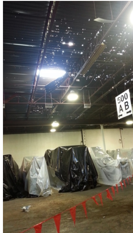
Case 13. Male roofer fell through a rusted metal roof deck approximately 22 feet to the concrete floor.
