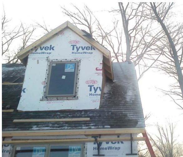
Case 14 . Male carpenter/roofer was working alone while installing shingles on a dormer on a 2-story house with a 10/12 roof pitch when he fell 9-15 feet.
