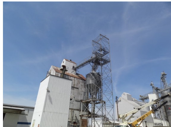
Case 24. Millwright fell 60 feet through an opening in a catwalk floor while disassembling and removing conveyor equipment from a grain elevator
