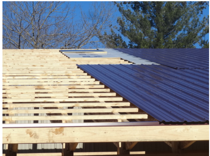
Case 25. Roofer fell 17-20 feet when walking down a purlin to obtain a piece of roof sheeting during the construction of a pole barn.
