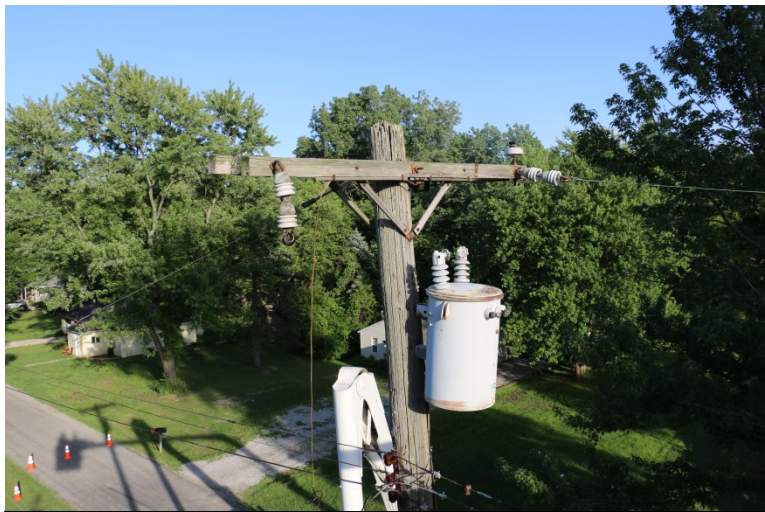
Case 19. Overhead lineman contacted an energized 13,280-volt overhead line.
