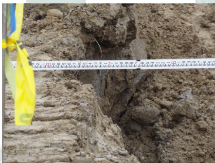
A male pipe layer in his 40s died in a trench wall collapse installing drain tile pipe. The trench had a 1½-foot seam of wet sand at its base and then 5 feet of wet clay. Falling clay forced a shovel to strike his right side, pinning him against the opposite side of the excavation.
