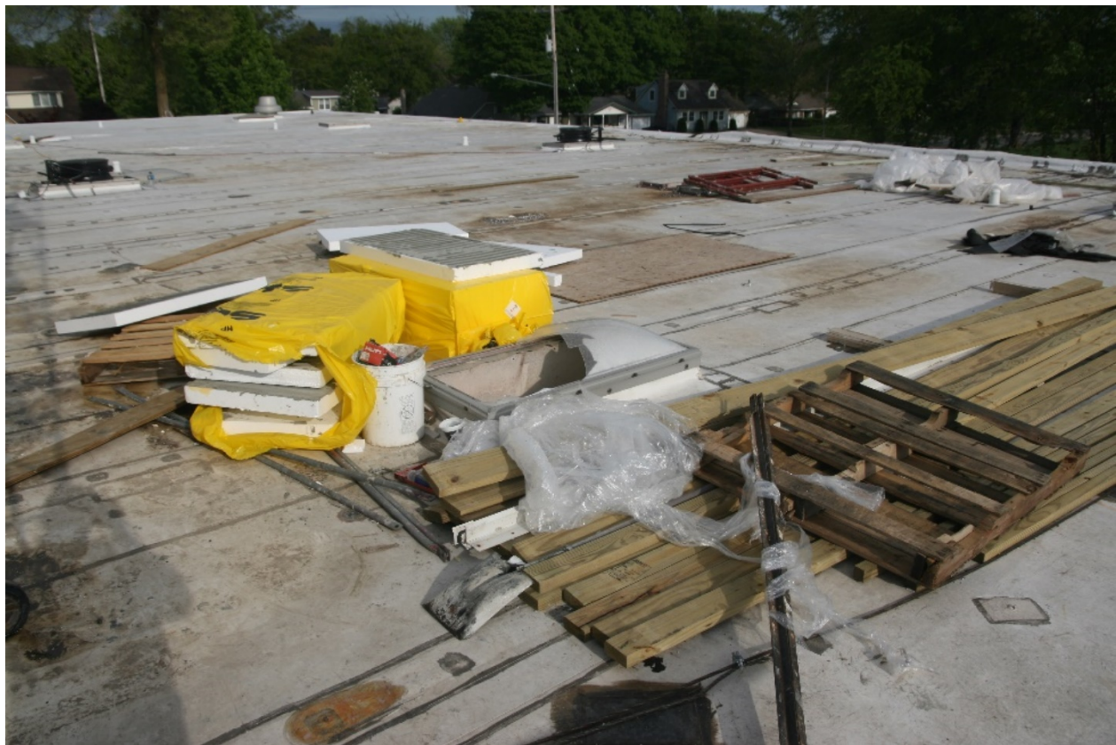
A plasterer/drywall installer died when he fell approximately 30 feet through a 24-inch by 48-inch plastic skylight. Narrative #29
