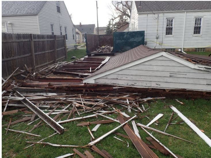
A laborer died when the roof of a carport/garage combination at a residential property being demolished fell onto him. Narrative #45
