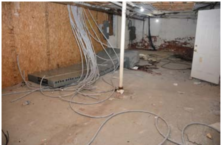
A journeyman electrician in his 60s died when a 40-gang meter bank and disconnect switch weighing approximately 700 pounds fell away from a wall and landed on top of him.
