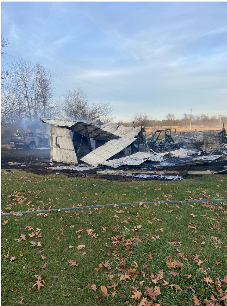
Case 5 . A male farmer in his 60s died due to asphyxiation due to smoke inhalation when he was caught under an electric golf cart that had caught fire during repair in a 20- by 40-foot metal pole barn/structure. Photo courtesy of responding police.
