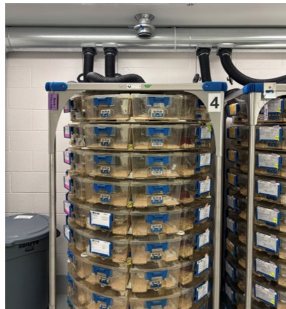
Figure 2. Plastic enclosures stacked on racks with air intake on outer edge of the rack. Air is pulled through the individual plastic enclosures to middle column and vented through ducts on the ceiling.
